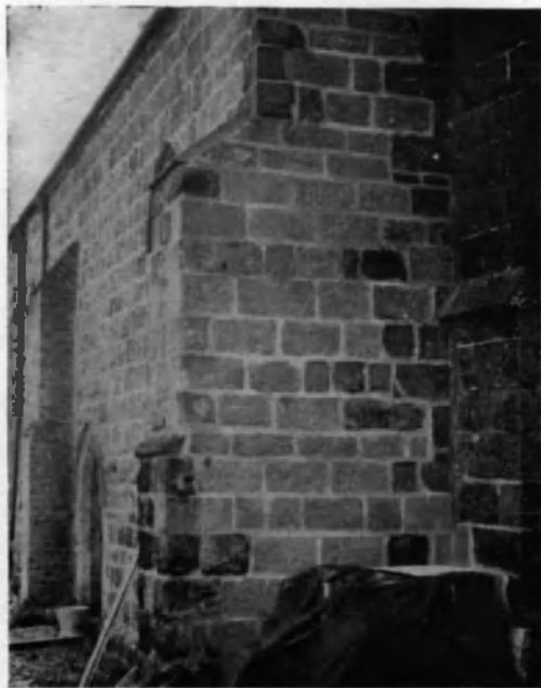
MALTBY CHURCH, LINCS., 1940. After Repair in 1940.
